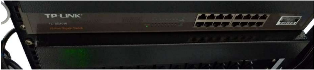
Figura 25 – Switch Gigabit TL-SG1016
